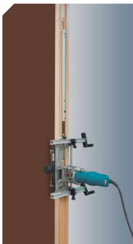
Making the second recess on the frame.
