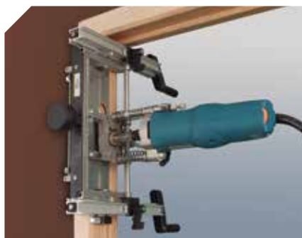
Making the upper recess on the frame.
